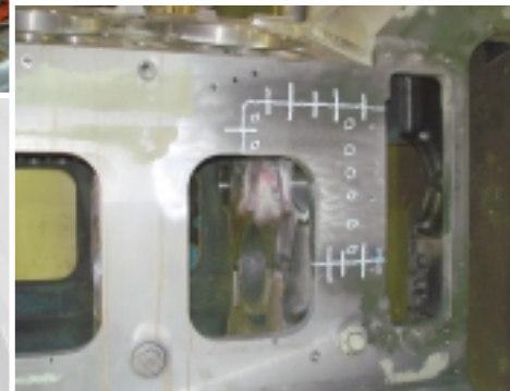
Repaired window section of 16 cylinder diesel generator, repair highlighted for clarity
