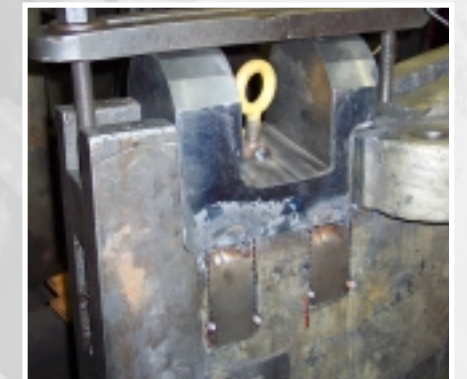
Broken press crown, metal locking repair in-process
