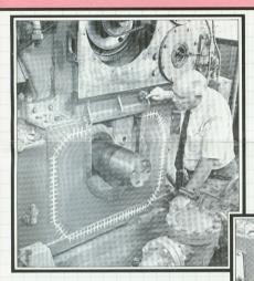
New cast iron section was cast, machined by Metal Locking to proper dimension and fit into prepared opening. It was then metal locked and sealed against pressure. This area has been highlighted to facilitate photography.
